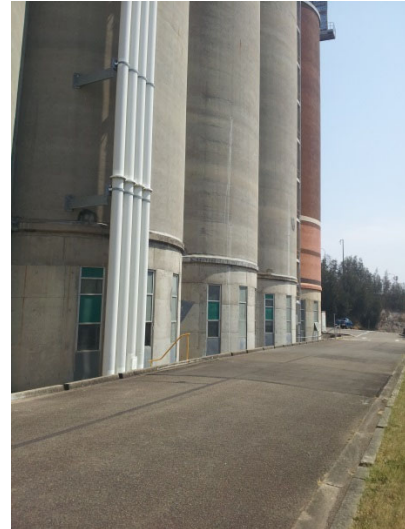
Silo 1212 & In-load pipes
